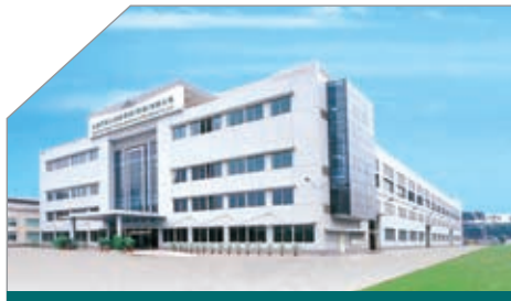
Monforts Fong's Manufacturing Plant, Shenzhen, China
