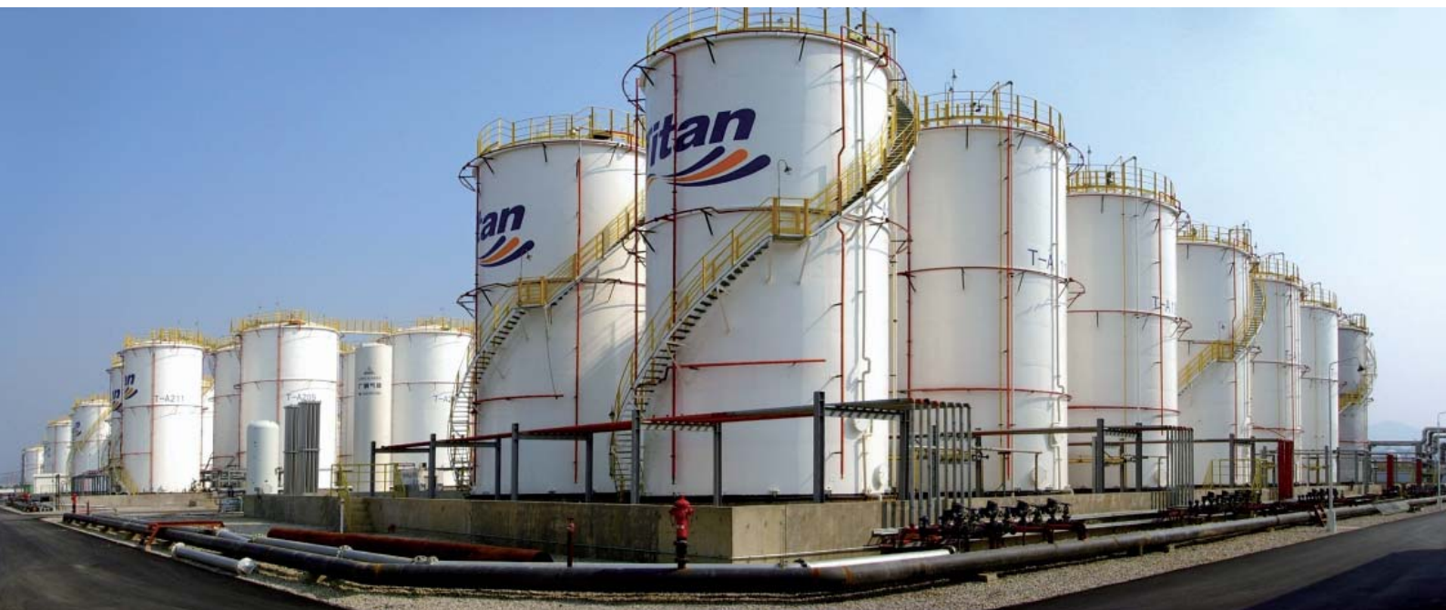
Nansha Phase II: Like Phase I, the facilities have been built to international standards and its advanced equipment, such as the Honeywell DCS system, ensures efficient and safe operations.
