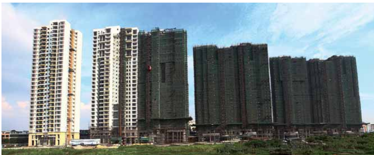
Imperial Garden – perspective (above); under construction (below)
