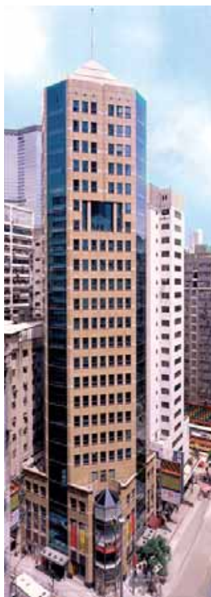
Chuang's Enterprises Building
