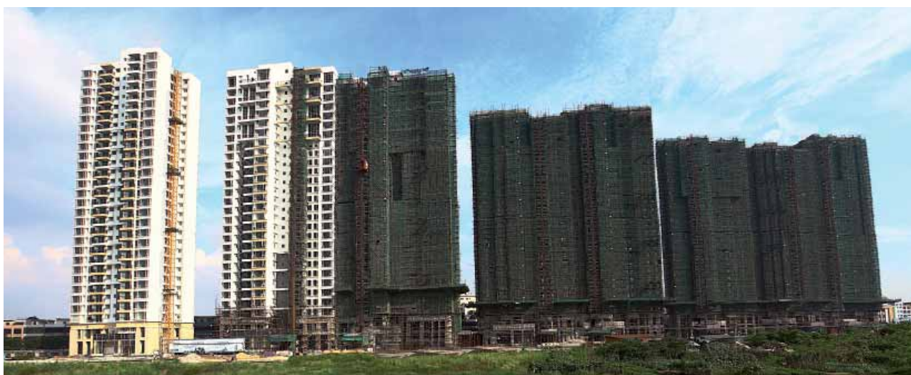
Imperial Garden – perspective (above); under construction (below)
