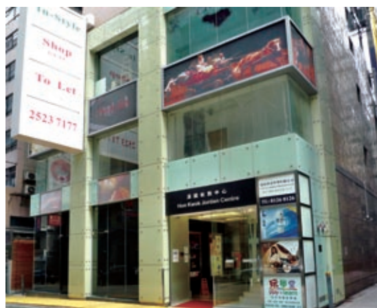
Hon Kwok Jordan Centre, Hillwood Road, Kowloon (One of the Group's investment properties in Hong Kong)
