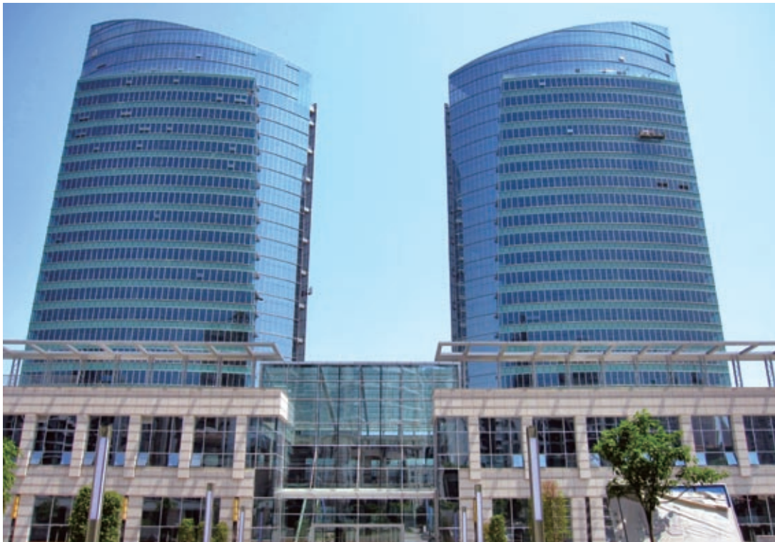
Chongqing Hon Kwok Centre, Chongqing (Construction works completed in March 2009)
