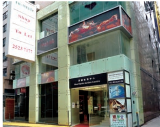
Hon Kwok Jordan Centre, Hillwood Road, Kowloon (One of the Group's investment properties in Hong Kong)
