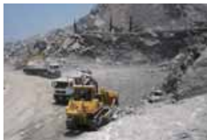
Quarrying and land reclamation project in Fujairah
