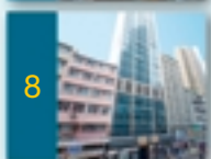
8 Yue Fai Commercial Centre Property Aberdeen, 42,751 sq.ft.
