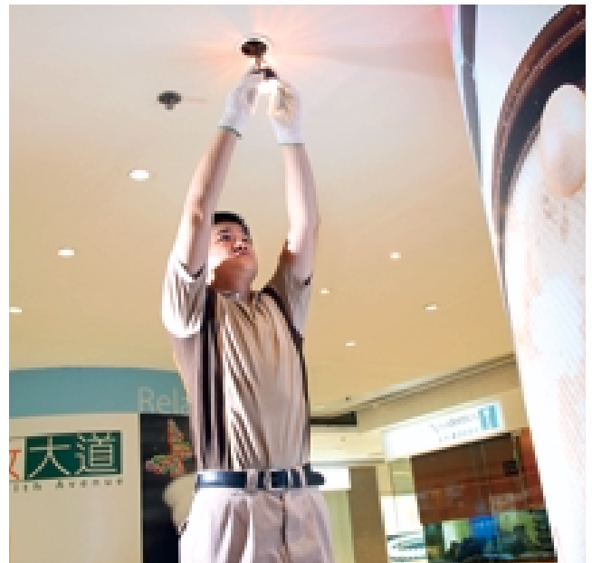
Installation of energy saving lighting device
