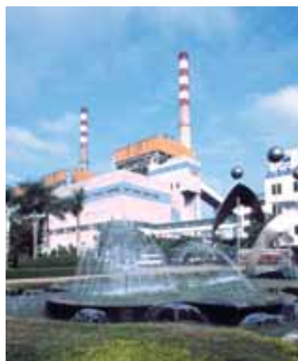
Zhujiang Power Plants
