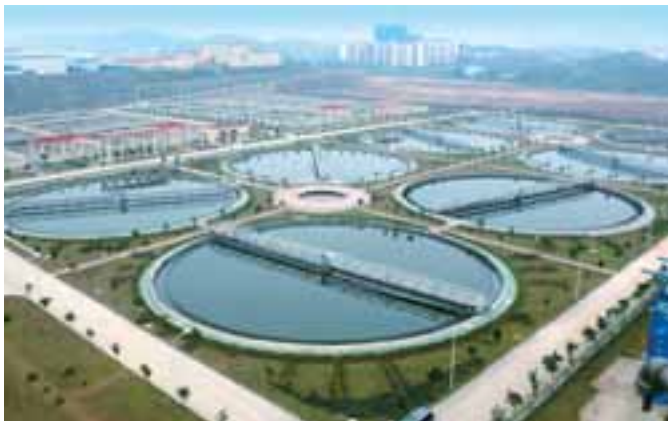
Chongqing Tangjiatuo Waste Water Plant
