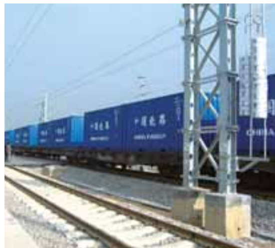
Kunming Rail Container Logistics Centre
