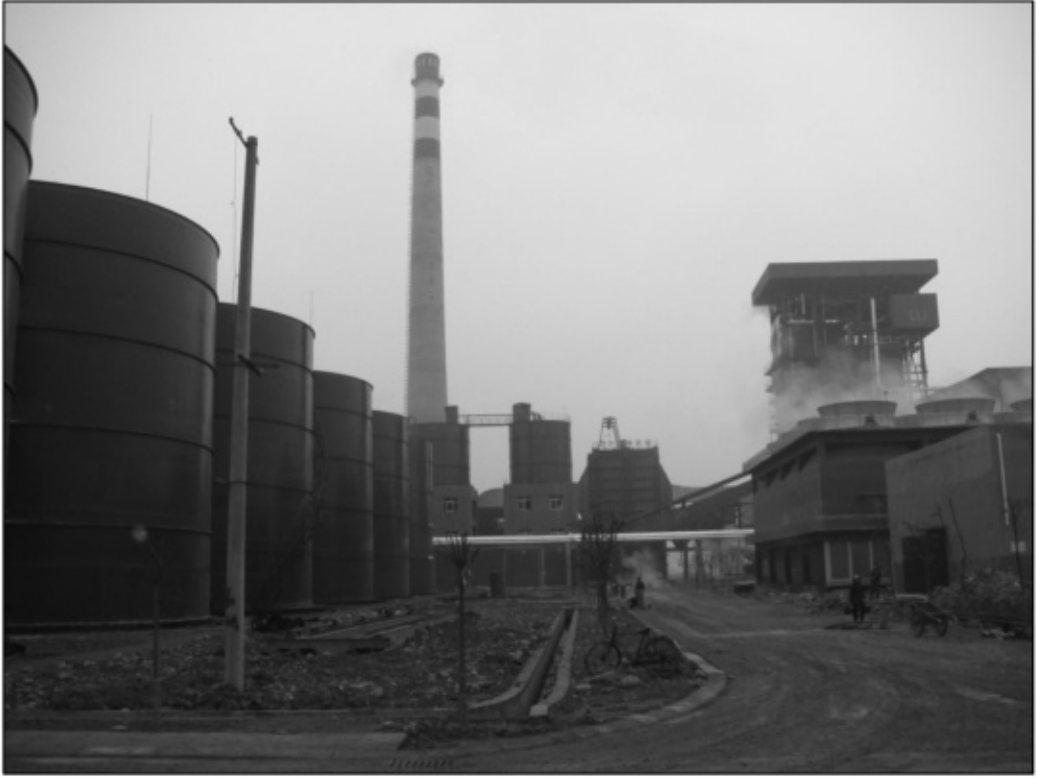
Power Plant/Water Treatment Facilities
