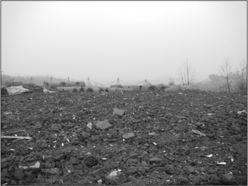
Surface Facilities Area (Prior Plants and Buildings Demolished)
