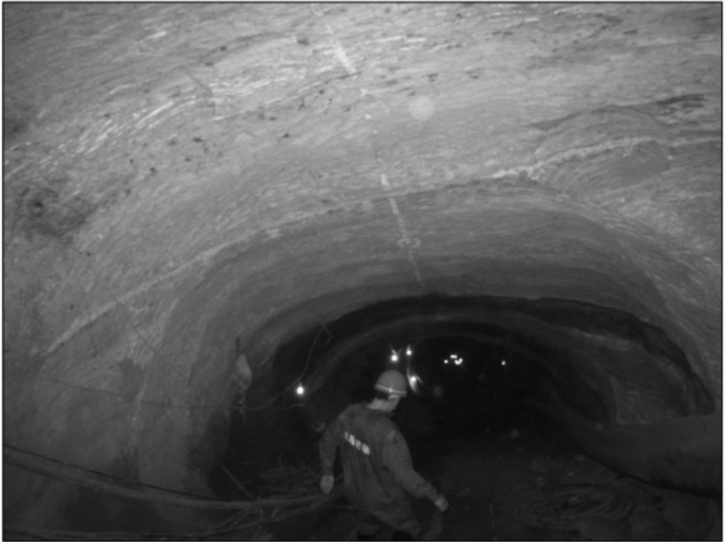
No. 3 Incline (developed by Roadheader)
