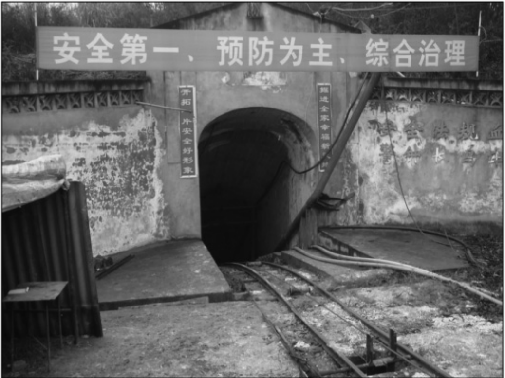
Entrance to Ore Hoisting Incline
