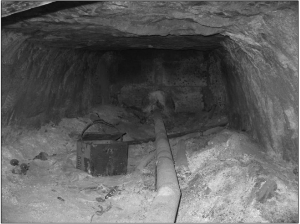
Solution Discharge Point for Abandoned Cell
