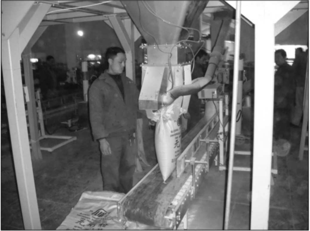
Processing Plant Bagging Area
