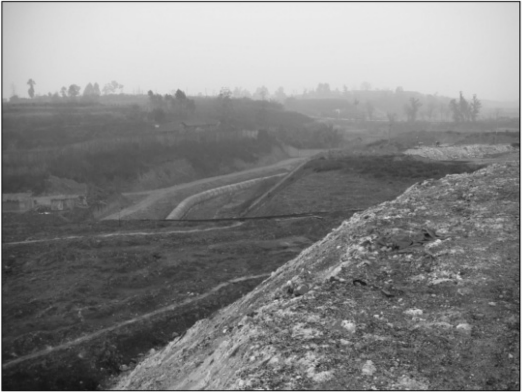
Site Preparation Area Valley Diversion Pipeline Construction
