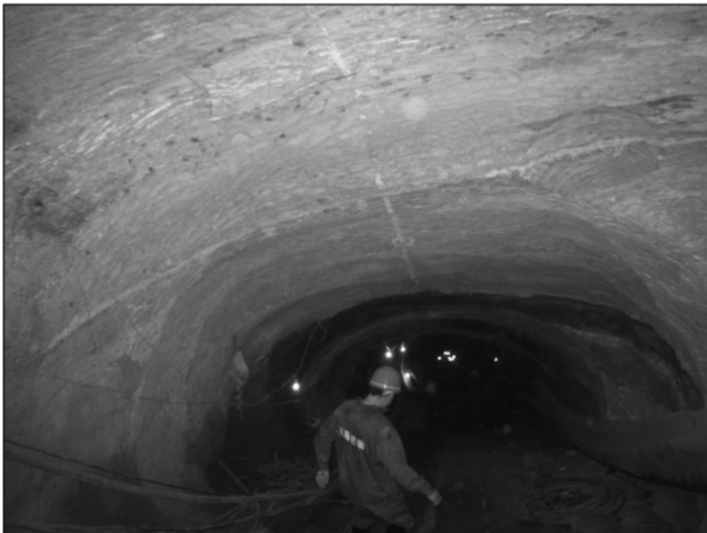
No. 3 Incline (developed by Roadheader)
