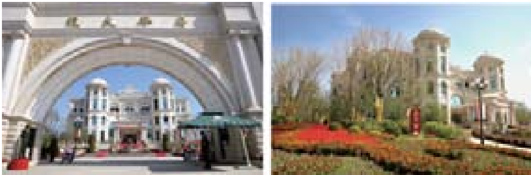
Clubhouse and Front Gate of Evergrande Palace Baotou Phase 1
