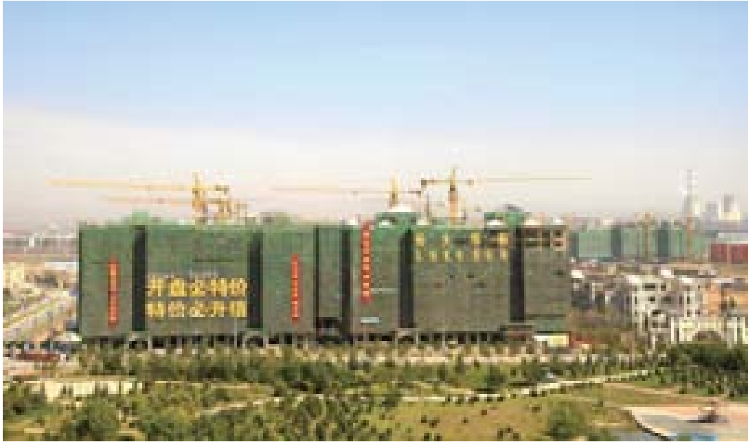
Construction Site of Evergrande Palace Baotou Phase 1
