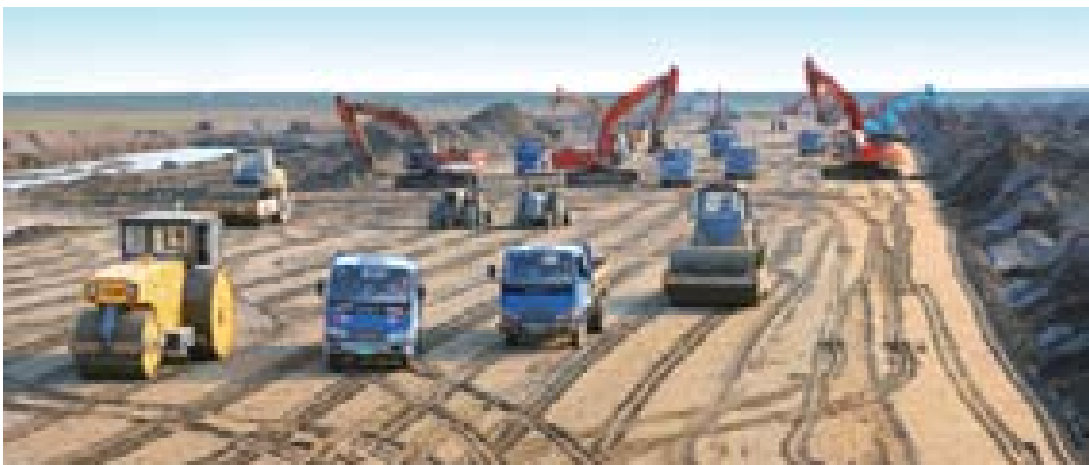
Road Construction site of Evergrande Splendor Qidong
