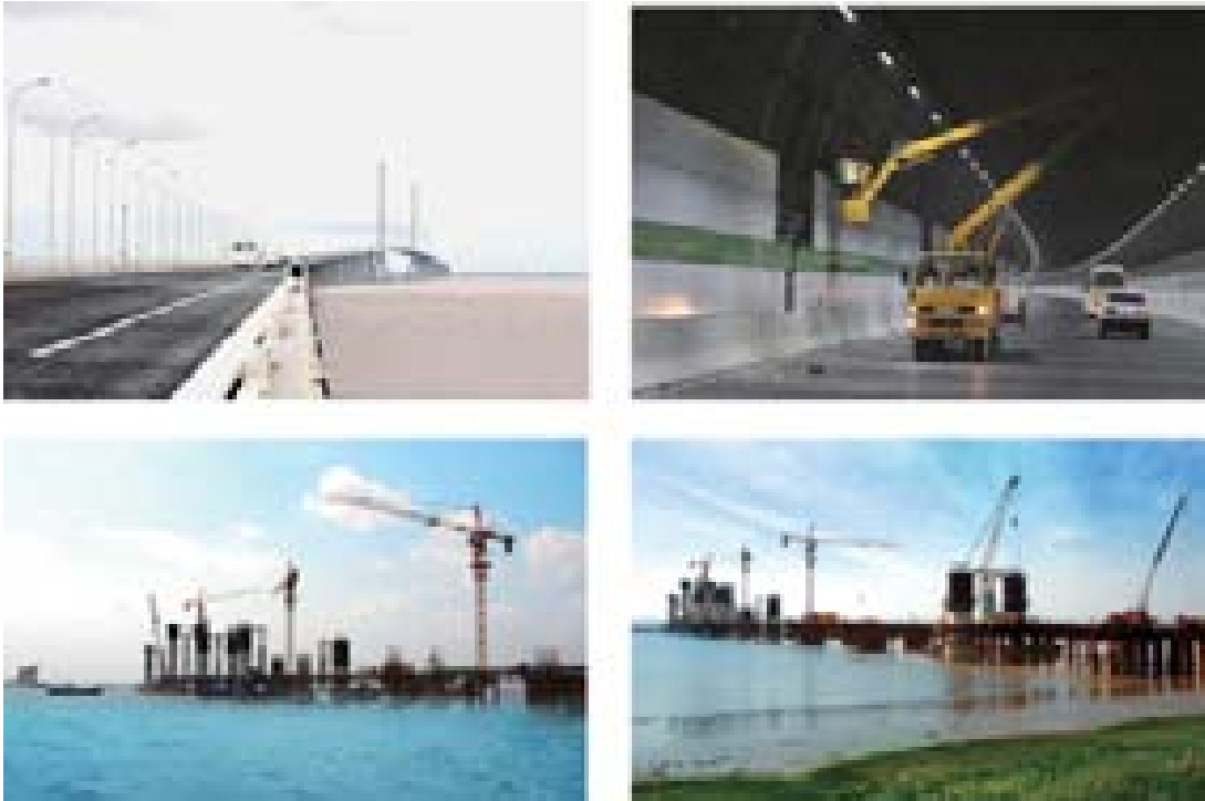
Construction Site of Shanghai-Chongming Island-Jiangsu Expressway
