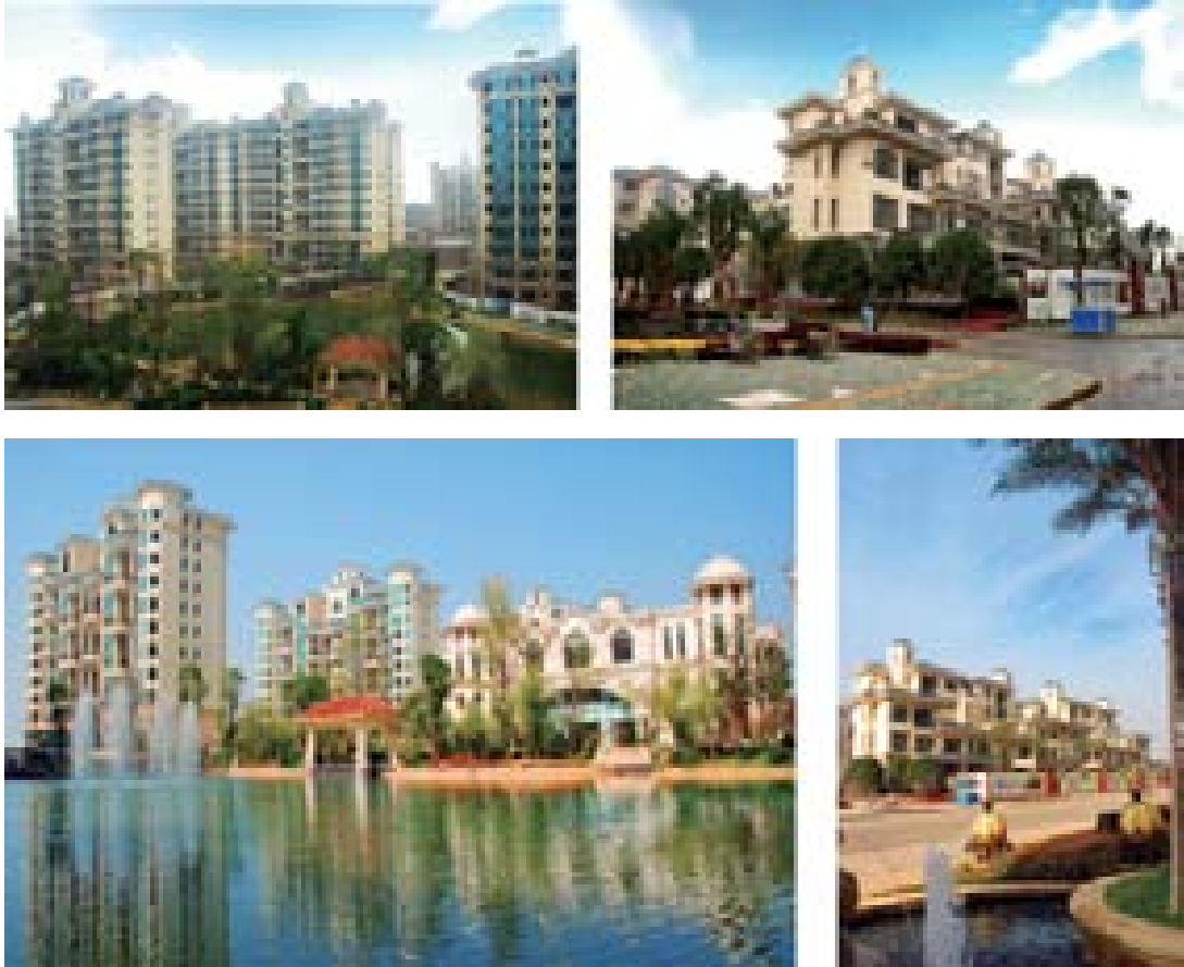
Construction Site of Evergrande Palace Wuhan Phase 1
