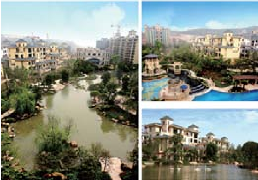
Garden View and Construction Site of Evergrande Palace Chongqing Phase 1
