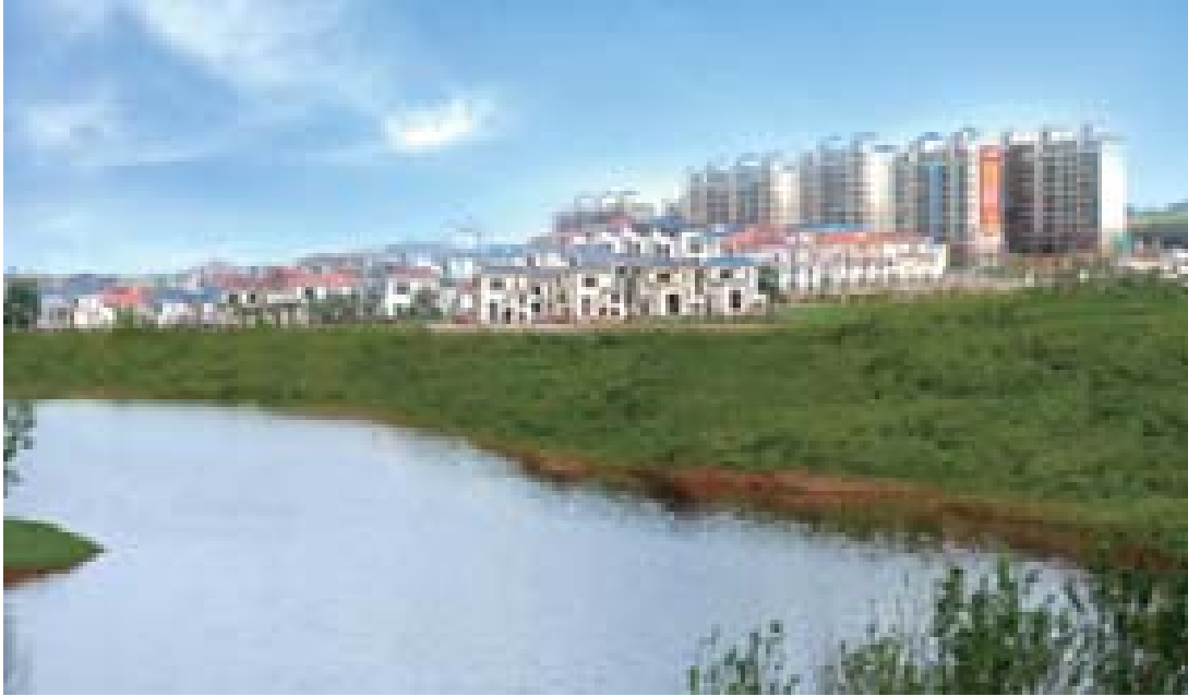
Construction Site of Evergrande Splendor Kunming Phase 1
