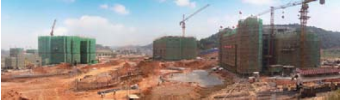
Construction Site of Evergrande City Changsha Phase 1
