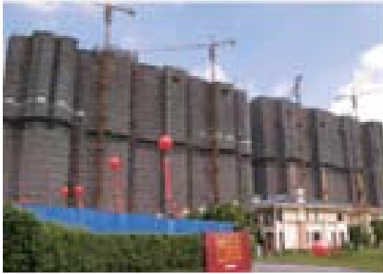
Construction Site of Evergrande Royal Scenic Peninsula Phase 2
