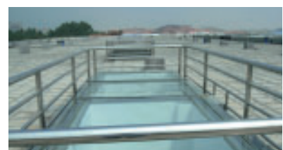
Skylights in the roof to illuminate the building using sunlight. 屋頂上利用太陽光為樓宇照明的光源。
