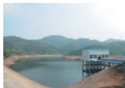
Water reservoir for factory in Huangjiang Dongguan PRC
