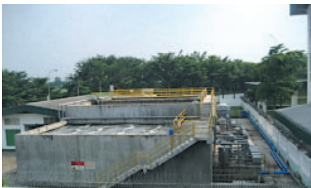
New water treatment facility at the factory that started operation in January 2009. (Dong Nai)
