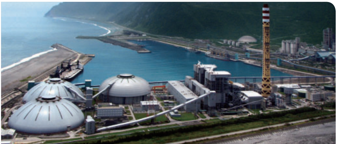
○ Ho-Ping Power Station, with repaired coal storage domes
