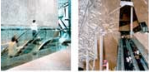
escalator to retail outlets at citibank plaza (left)
