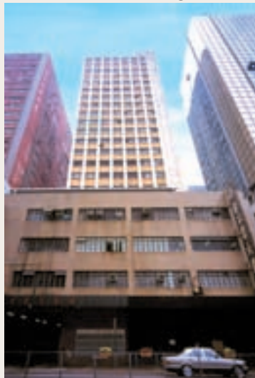
Bonsun Industrial Building
