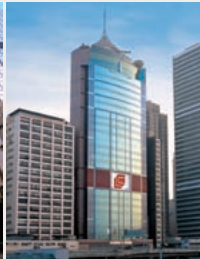
Western Harbour Centre
