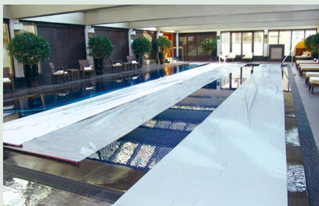
Laying the pool cover at The Peninsula Beijing to reduce water and heat loss and thereby save on water and energy consumption.
