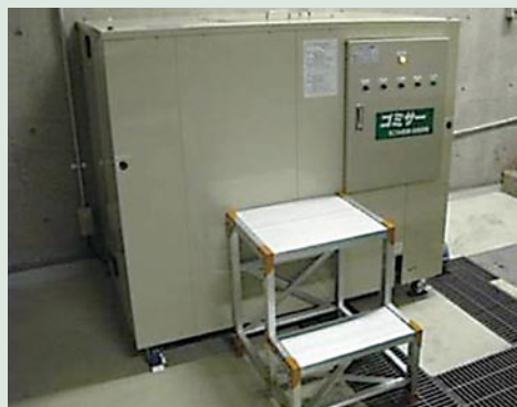
The Peninsula Tokyo introduced the 'Gomizer' machine in 2009, which converts perishable waste through a cost effective, environmentally responsible yeast/bacteria process into a liquid for safe discharge to the sewage system, thereby dispensing of more than 50 kg of waste per day. As of 1 March 2009, an estimated 15,000 kg of perishable garbage had been processed.
