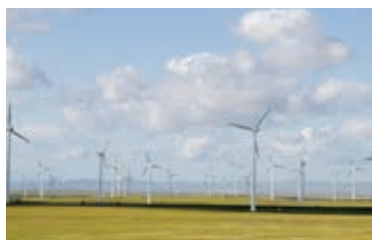
Xilingol Guotai Wind Power Plant
