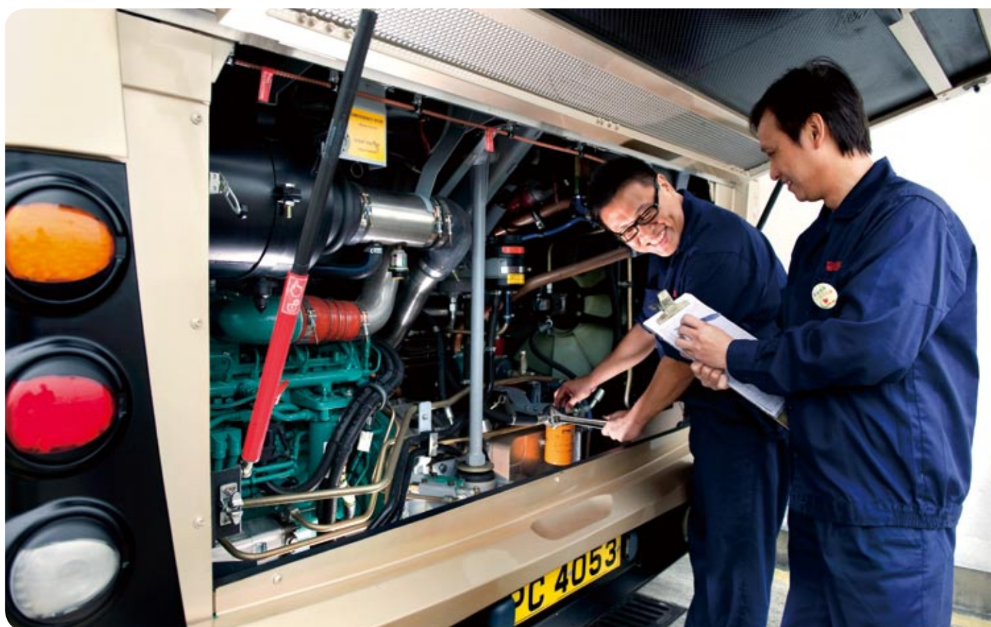
A rigorous maintenance regime is the key to our safe and reliable bus services
