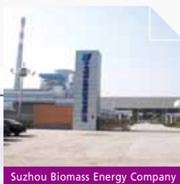
Suzhou Biomass Energy Company
