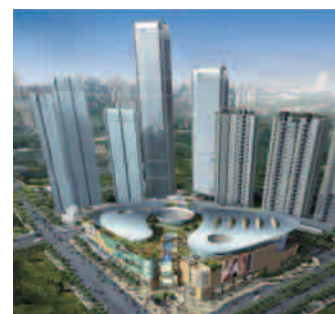
Curtain wall construction project — Hangzhou MIXC
