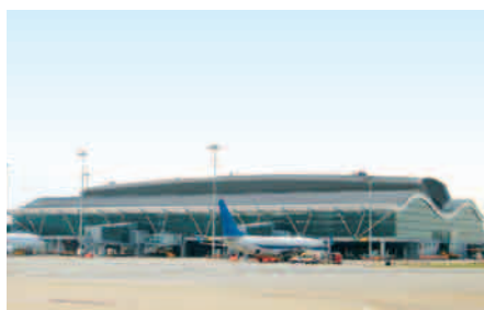
Curtain wall construction project — North Satellite Concourse, Hong Kong International Airport
