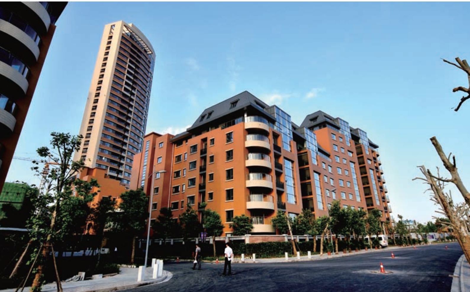
The Riverview Phase 1 at Wuhan Tiandi
