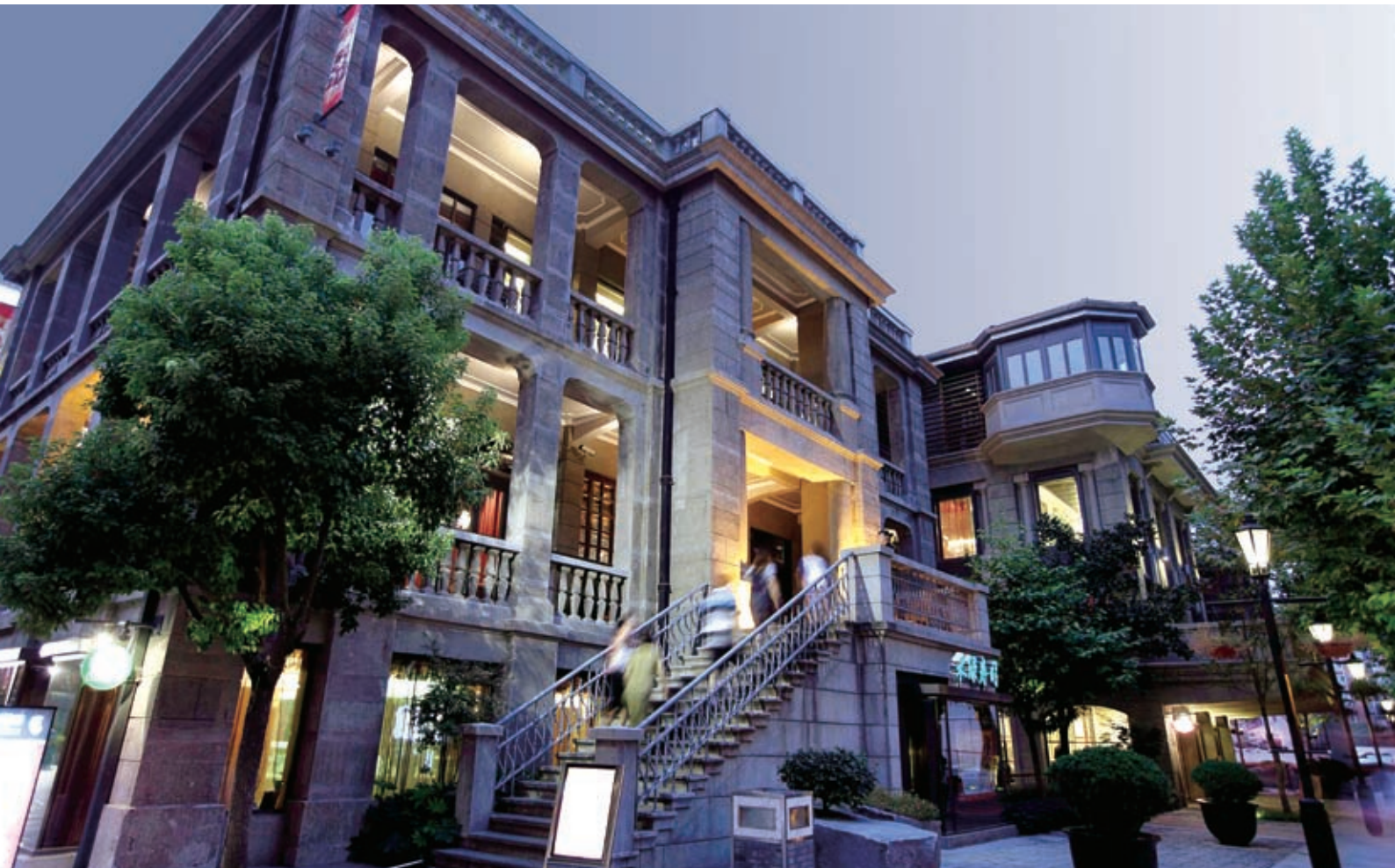
Commercial properties at Wuhan Tiandi
