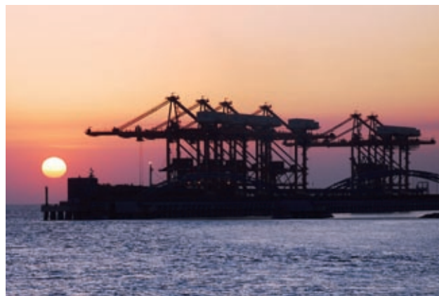
Caofeidian 250,000-ton class Ore Terminal
