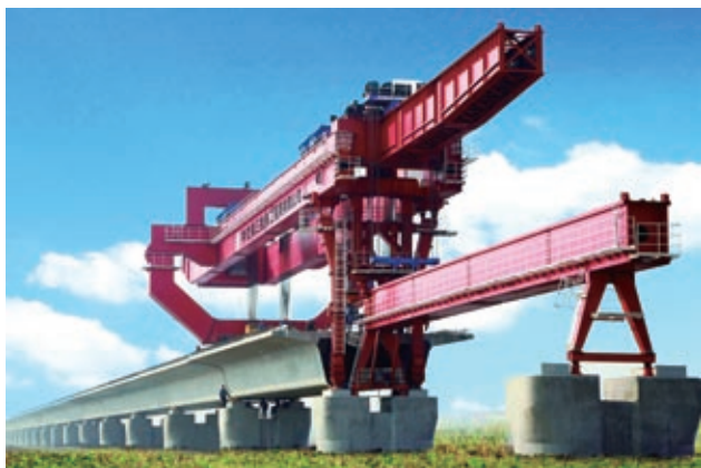
Harbin-Dalian PDL under construction
