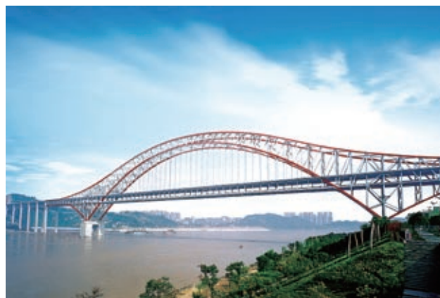
Chaotianmen Yangtze River Bridge, a steel arch bridge with the longest span of steel-box girder in the world
