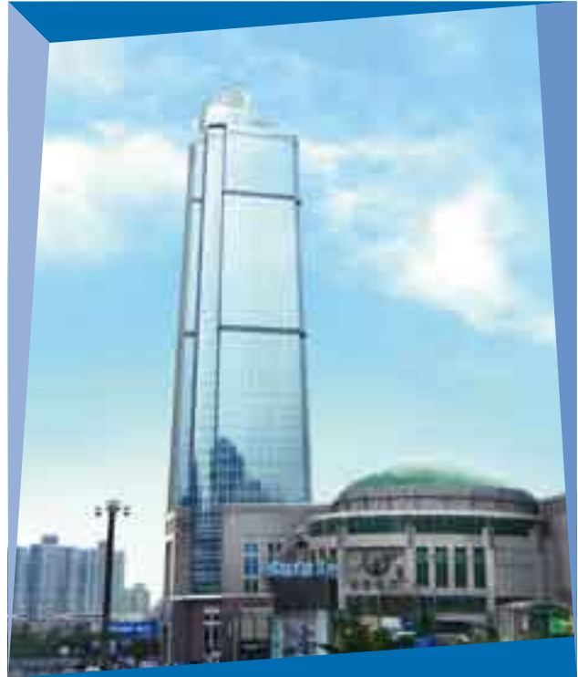
Office Tower II, The Grand Gateway, Shanghai
