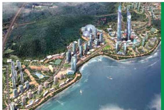
Infrastructural construction works at Woonbook Project in Incheon Free Economic Zone, Korea are in progress
