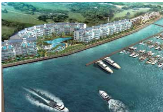
Marina Collection, a property development project at Sentosa Cove, Sentosa Island, Singapore
