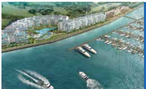
Marina Collection, a property development project at Sentosa Cove, Sentosa Island, Singapore
