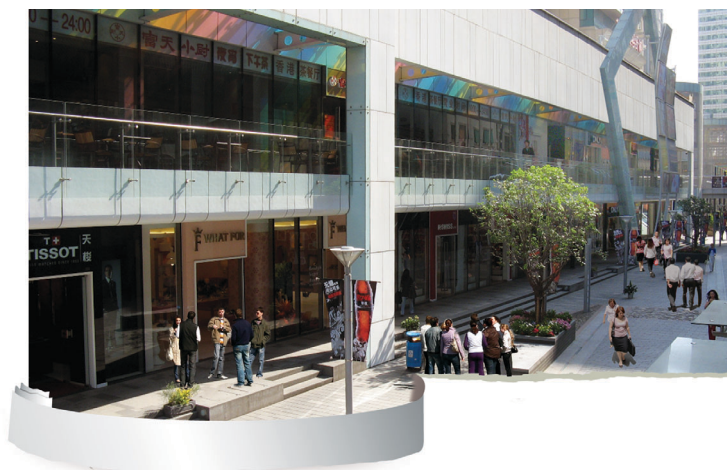
In Point, 169 Wujiang Road, Shanghai
