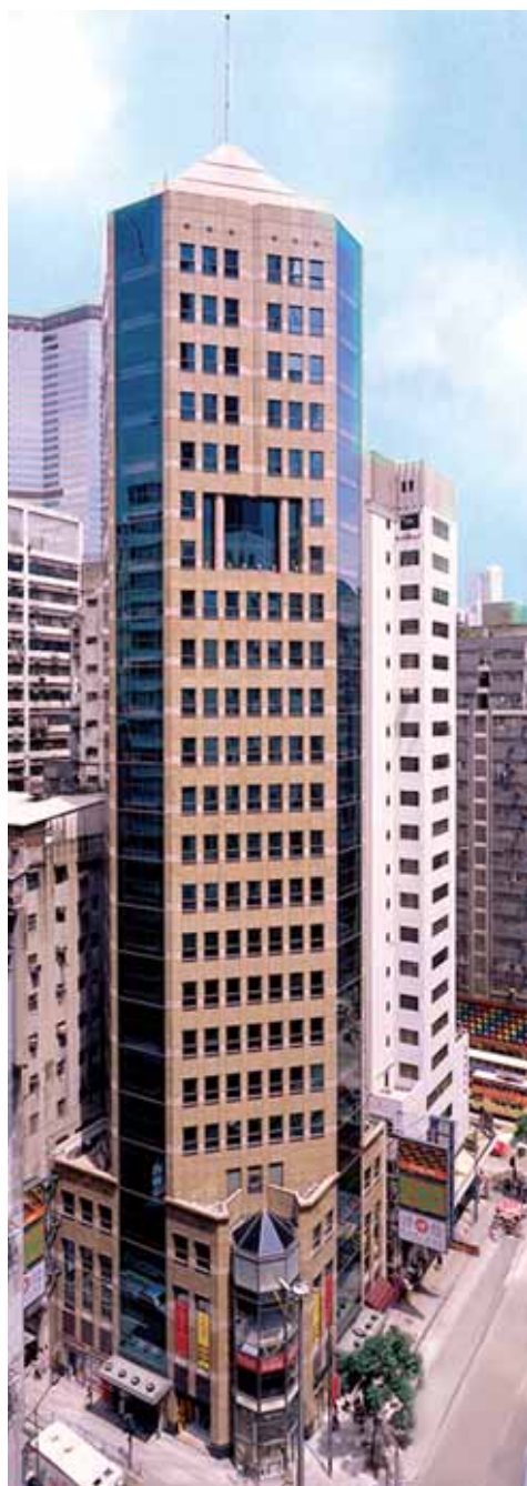
Chuang's Enterprises Building
