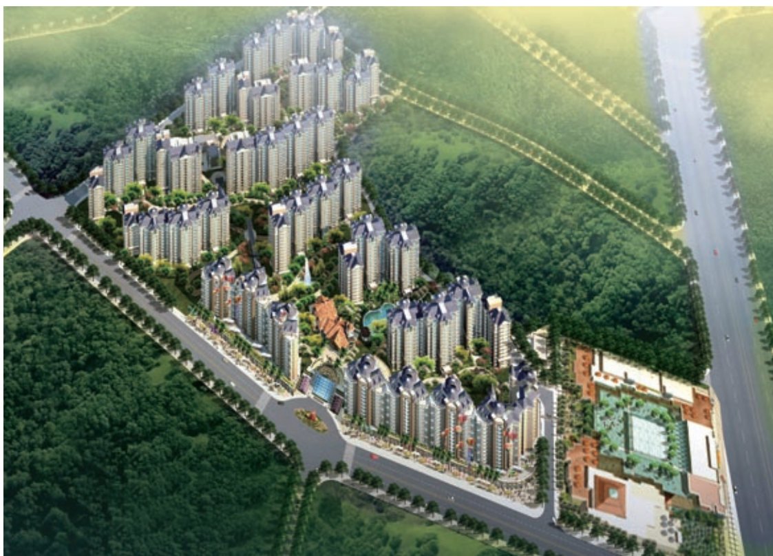
Botanica development project, Tian He District, Guangzhou – Architect Perspective
