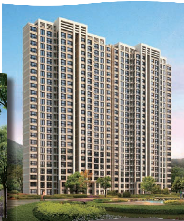
Residential apartments in Greenville, Dalian Tiandi
