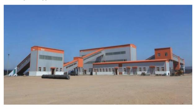
The coal processing plant at Ceke uses a dry separation process and had a processing capacity of 1.2 mtpa as at 30 June 2010. Since its completion of construction in December 2009, we have commenced our trial operation at the coal processing plant at Ceke and are currently in the final stage of testing and fine tuning the production line.
