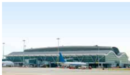
Curtain wall construction project — North Satellite Concourse, Hong Kong International Airport
