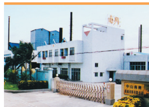
Front View of the Industrial Laminate Plant in Zhongshan, the PRC
