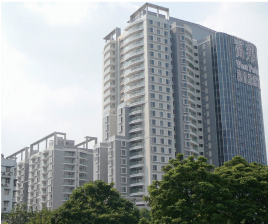
Guangzhou West Point
