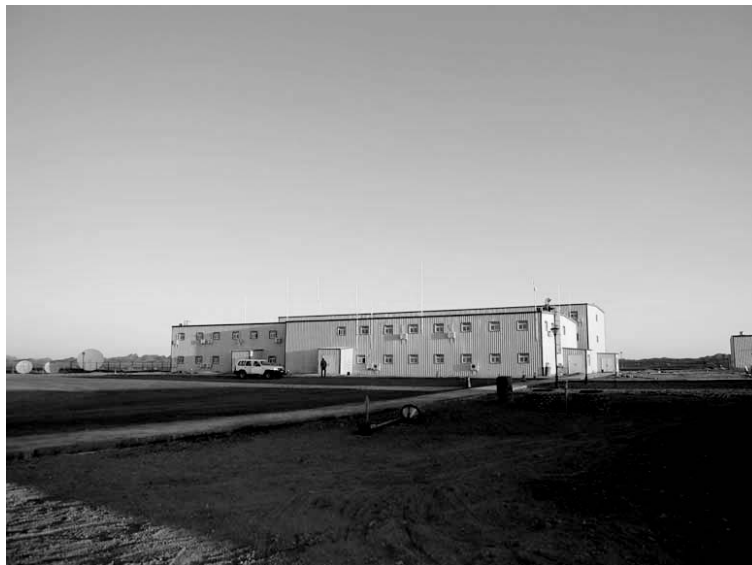
Photo 25.2 Permanent 'Man-Camp' Facility
