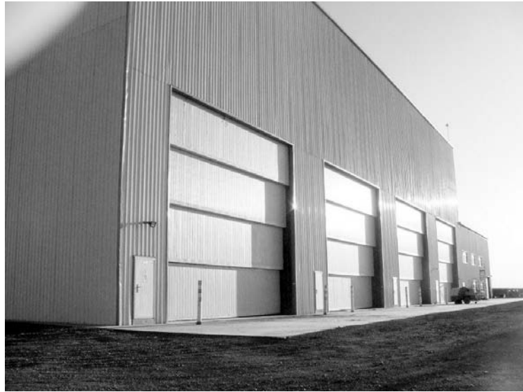
Photo 25.1 Permanent Maintenance Facility
