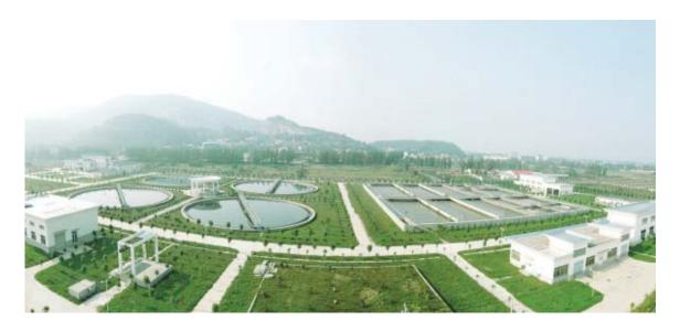
The project, located in Xiangcheng District of Xiangfan City, Hubei Province, involved the design and construction of a wastewater treatment facility with a wastewater treatment capacity of 100,000 tonnes per day. The treatment process adopts the A<sup>2</sup>/O pre-denitrification technique.
