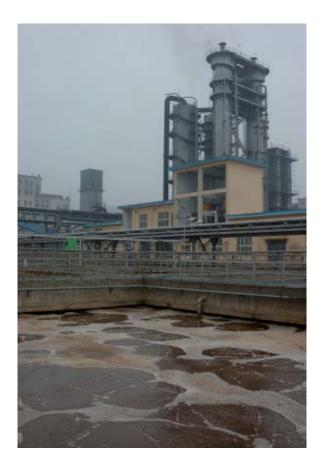
The industrial wastewater project in Handan City, Hebei Province, adopts the physical-chemical treatment technique utilizing a high efficiency settling pond with mud external enhanced flocculation functions, tube settling technology and mud concentration, a high efficiency lime-softening settling pond and a V-shape filtering pond. The project has a treatment capacity of 3,000 tonnes per hour.
