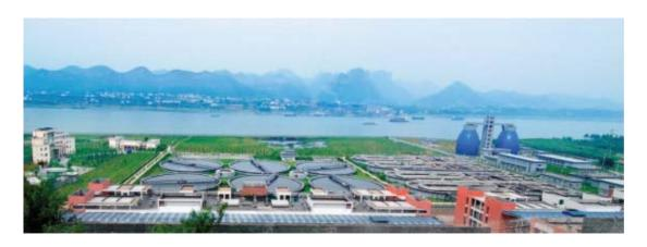
The project involved the design and construction of a 440,000 tonnes/day water treatment facility, a 200,000 tonnes/day wastewater treatment facility and laying part of the pipeline network system of Yichang City, Hubei Province. The water treatment plant provides tap water for the entire city of Yichang, which has a population of more than 4 million.
