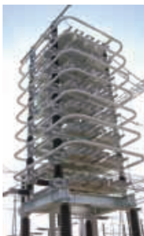
HV power capacitors
