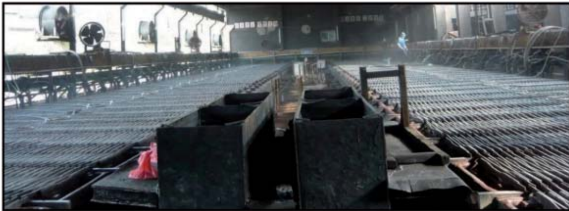
Figure 6-11: Electrolysis Shop at Start Electrolysis Plant
