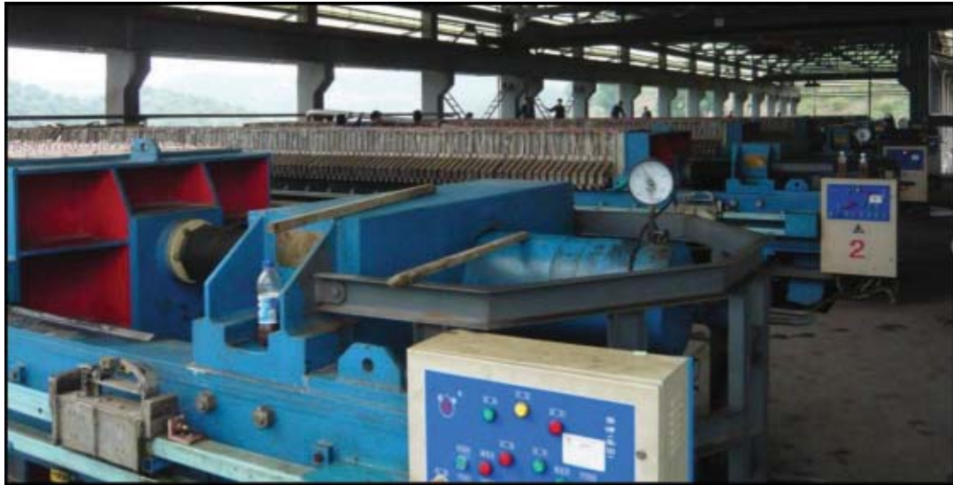
Figure 6-10: Press Filtration Shop at Tiangong Electrolysis Manganese Plant
