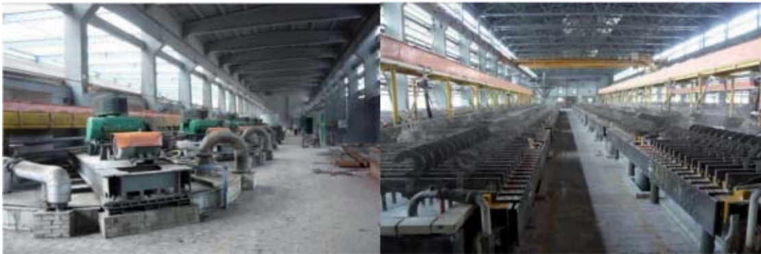
Figure 6-14: An Overview of Chemical and Electrolysis Workshop
