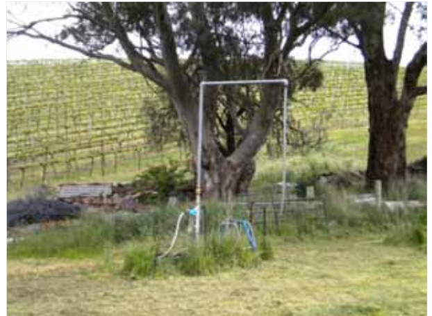
Overhead filling point
