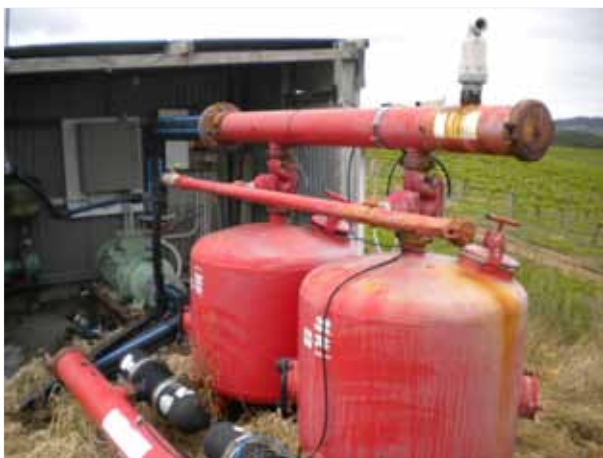
Pumping and filtration infrastructure
