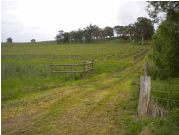
Causeway across winter creek
