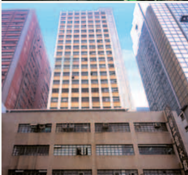
Bonsun Industrial Building
