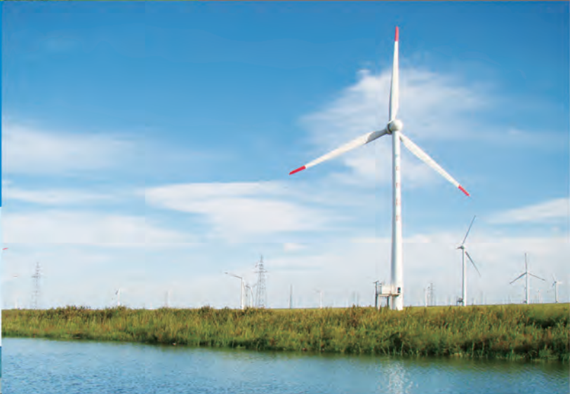
▲ China Power Dafeng Wind Power Project
