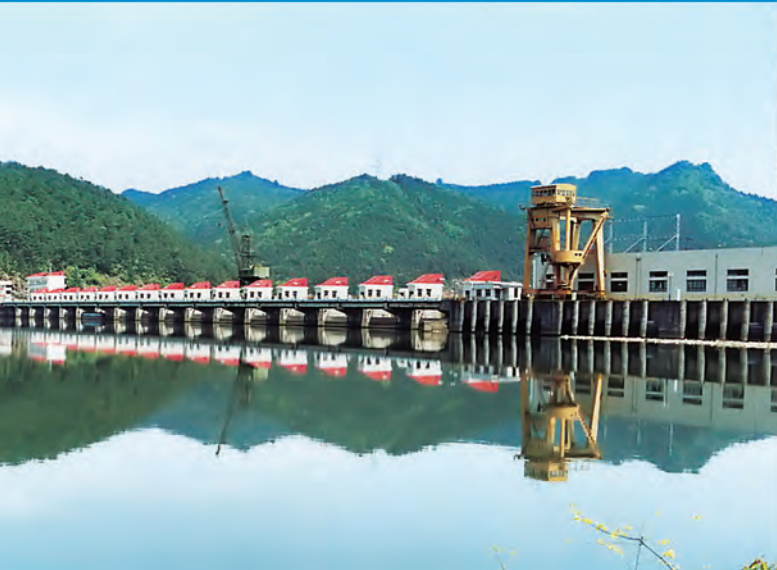
▼ Fujian Shaxikou Hydro-electric Power Plant
