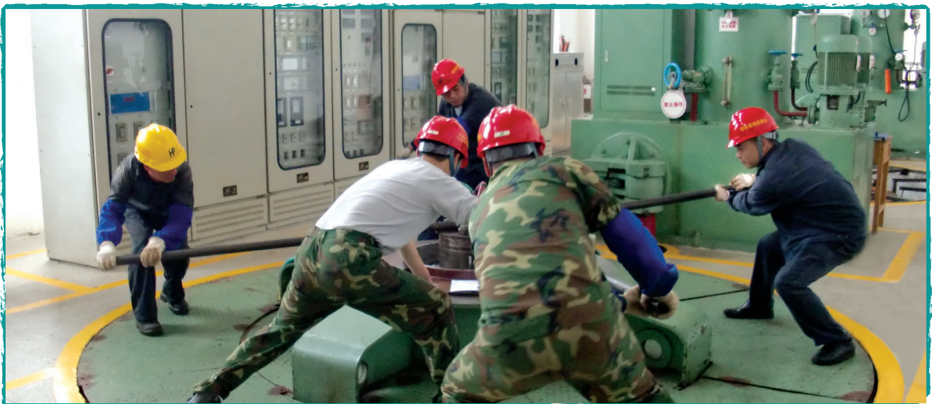
Teamwork at one of the Huaiji hydropower stations
