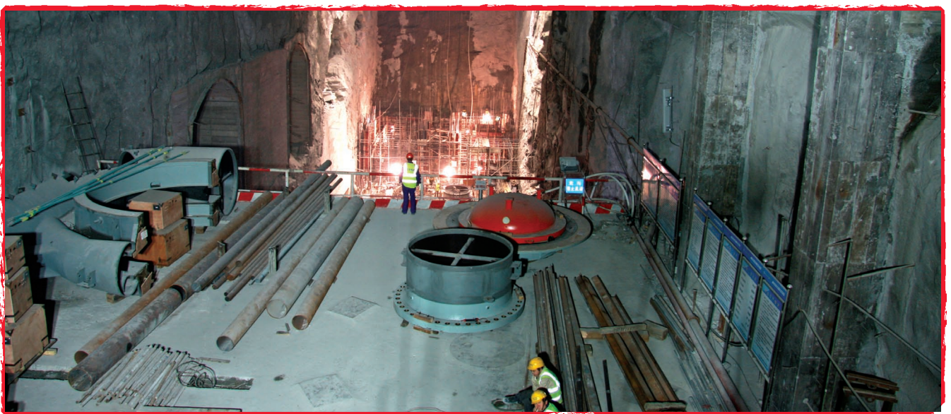
Underground power house construction at our Jiangbian hydro project
