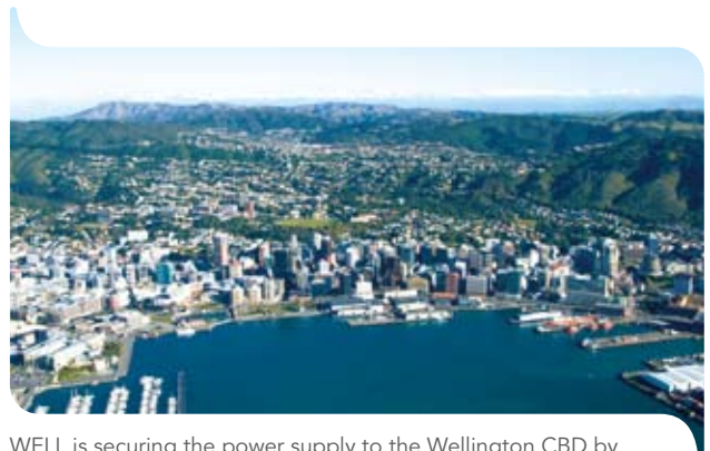
WELL is securing the power supply to the Wellington CBD by replacing 5 km of sub-transmission cable.
