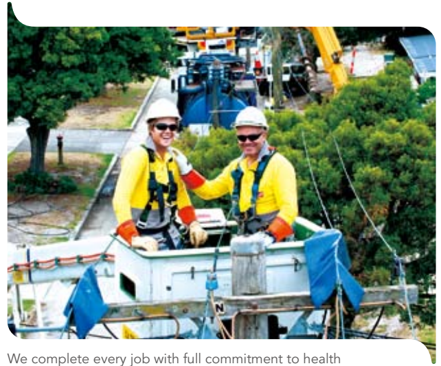
We complete every job with full commitment to health and safety.
