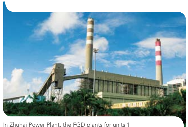
In Zhuhai Power Plant, the FGD plants for units 1 and 2 have been operating smoothly.
