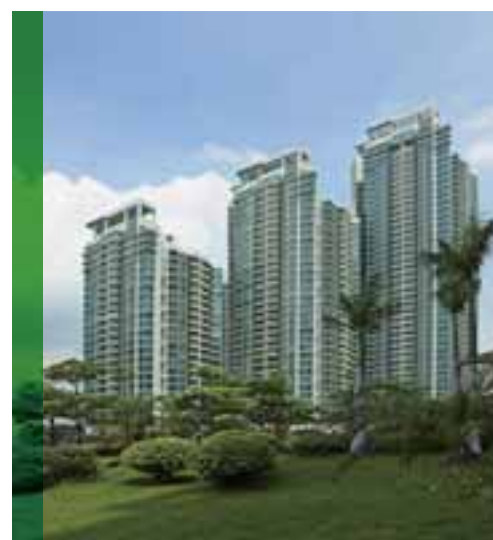
The last two 50-storey towers of Guangzhou The Riverside, located above Huangsha Metro overlooking the splendid views of the Pearl River.
