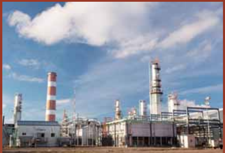
Husky Energy's Ram River Gas Plant, Canada.
