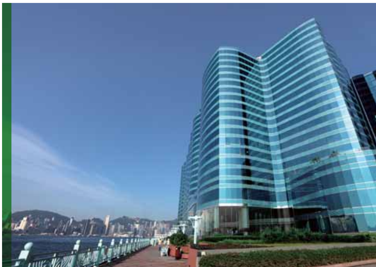
Located along the scenic waterfront of Victoria Harbour, the office towers of The Harbourfront offer a spectacular view of Hong Kong Island's skyline.
