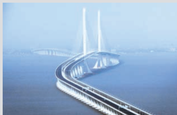
Shanghai Yangtze River Tunnel Connection Project
