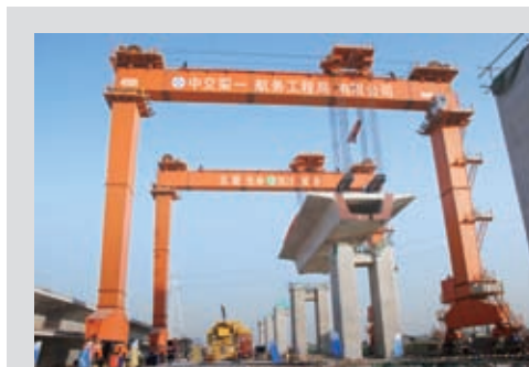
Beijing-Shanghai High-Speed Railway under construction
