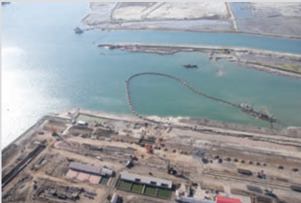
Jingtang Port 200,000t-class navigation channel dredging
