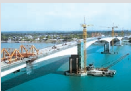
Mekong River Bridge in Cambodia
