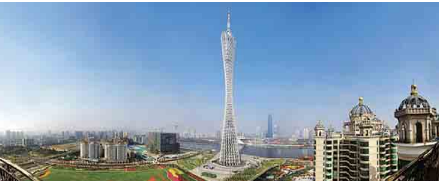
Guangzhou Regal Riviera is located next to the Guangzhou TV Tower 毗鄰廣州電視觀光塔的廣州珠江帝景
