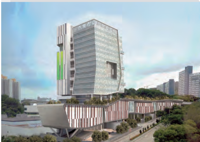
New Academic and Administration Building at City University of Hong Kong 香港城市大學新教學及行政大樓
