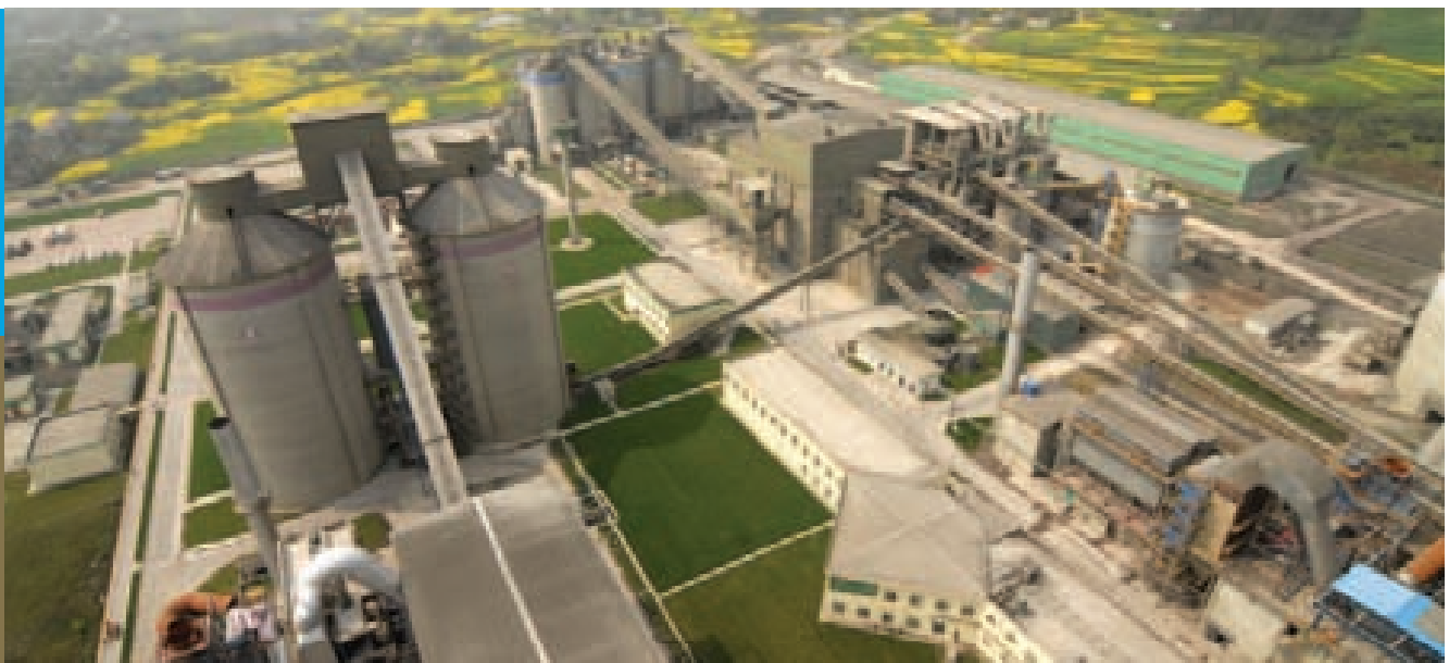
LSOC continues to reduce energy consumption and enhance operational efficiency
