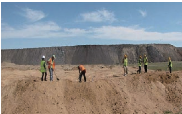
Field cultivation activities after grading by a dozer
