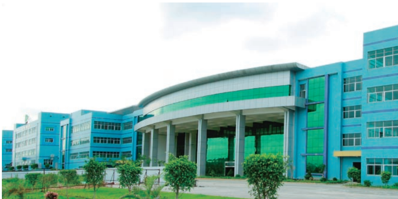
Outlook of the composite office building of Yuquan plant in Fenggang 鳳崗玉泉廠房綜合辦公樓之外貌
